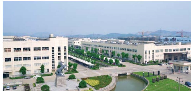
Yuyao Production Base Built in 1984 Kitchen appliance production base Electric water heater production base
